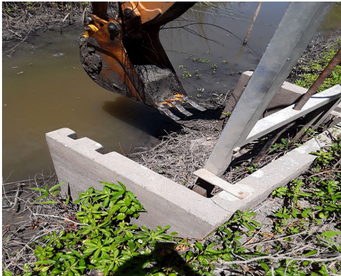
Image: cleaning water control structure
