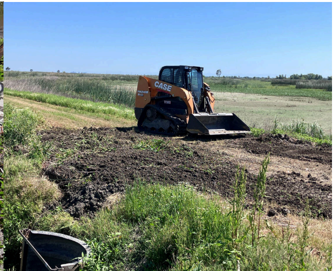
Image: repairing damages culverts
