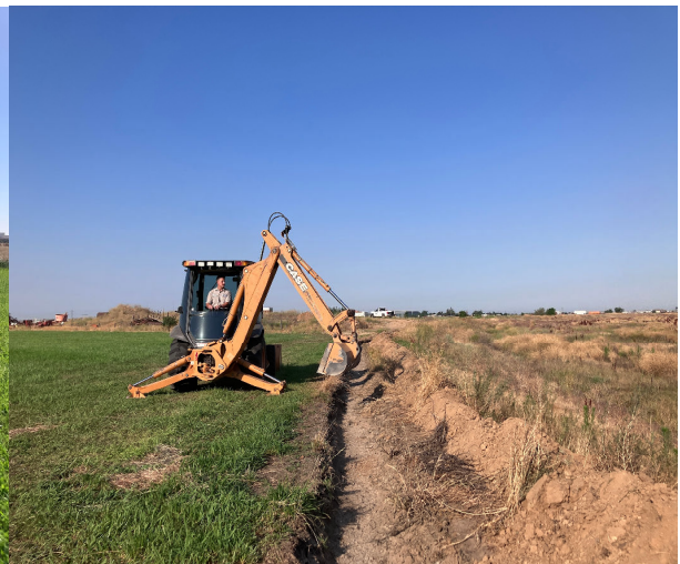
Image: Reinforcing levee
