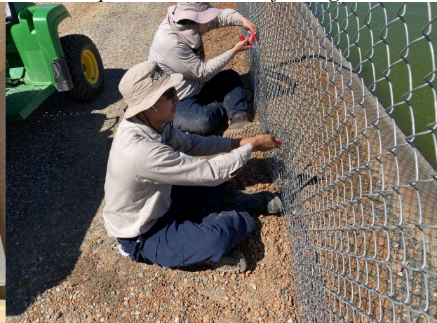
Bottom Right: Picture of technicians installing additional predator exclusion fencing.
