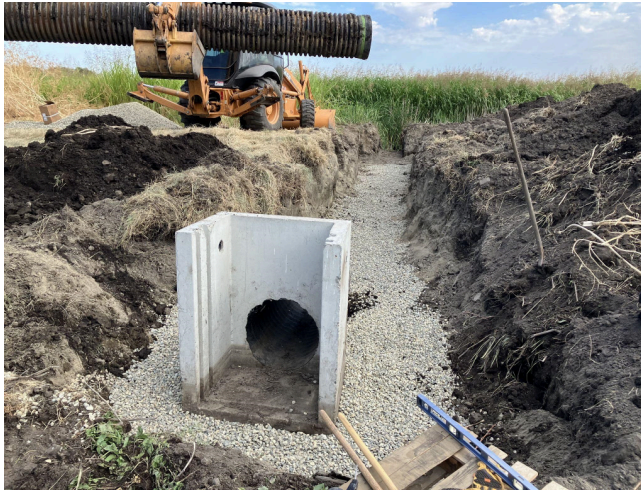
Image: Excavation and Installation
