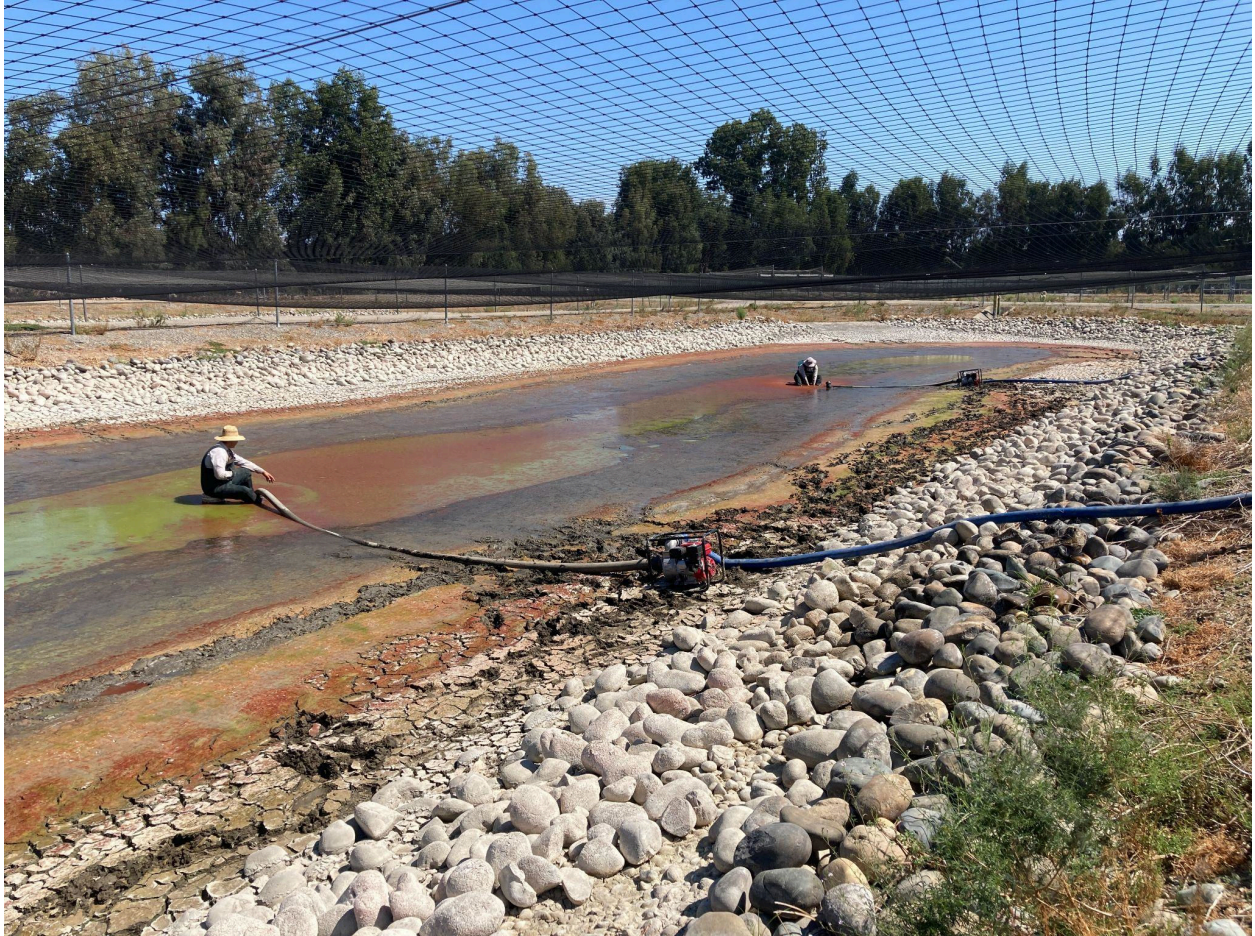
Above : Picture of technicians draining a pond down.
