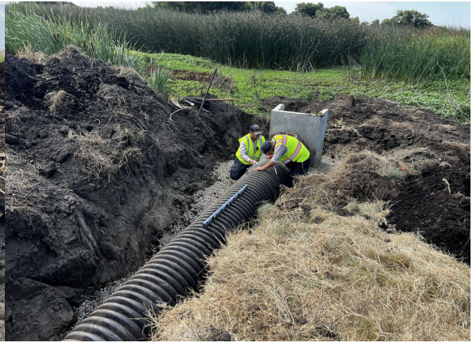
Image: Reseating pipe to control structure
